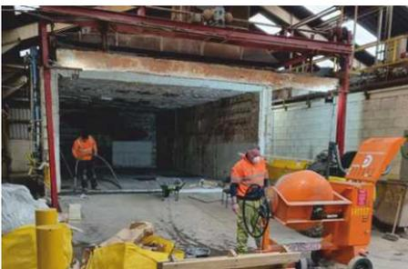
Our clay division refurbished one of our 2 intermittent kilns at Cawthorne; the kiln is used in Denlok jacking pipe production
