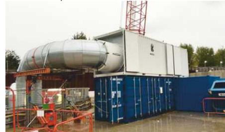
Gainsborough supplied HS2's Victoria Road tunnelling site with a temporary ventilation system
