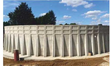
We supplied 4.3m high Sealwall precast sectional tank units to a waste water project in Norfolk
