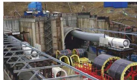
Wombwell & Gainsborough also joined forces to produce a complete temporary ventilation package for the West Ruislip to Euston HS2 sections
